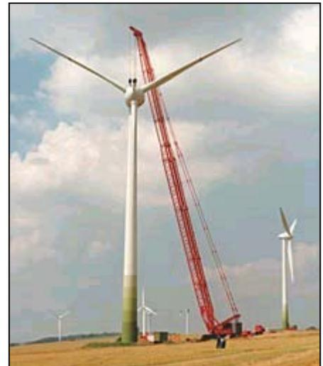
A Liebherr LR 1400/1 crawler crane lifts a 38 metric ton propeller 70 m for installation at a wind power plant in Dorntal, Germany. Normally two cranes lift and manipulate the propeller from horizontal to vertical, but in this case the task was accomplished with a single specially rigged crane. (Photo courtesy of Liebherr-Werks Ehingen GmbH.)
